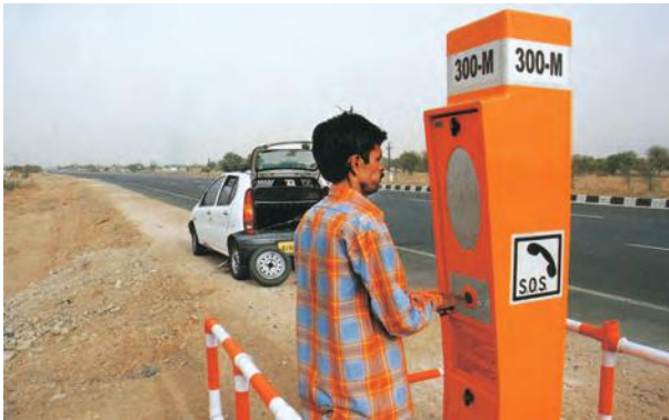
Fig.7.10 : Emergency call box on NH-8
