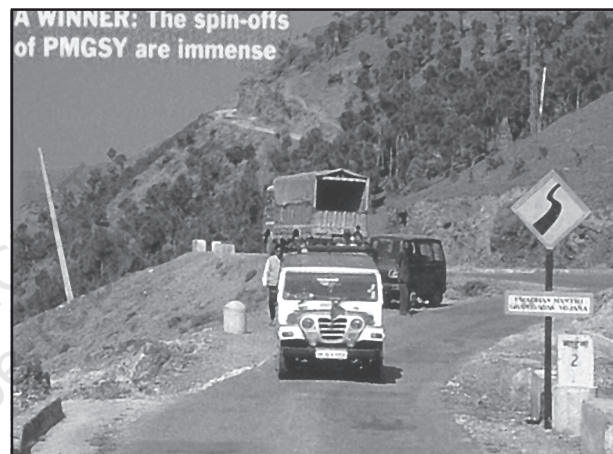
Fig. 10.2 : Road constructed under the Pradhan Mantri Gram Sadak Yojna
