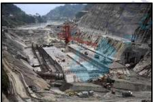
Lower Subansiri Hydroelectric Project (LSHP) is a 2000 MW run-of-the-river project on the Subansiri River, on the Arunachal Pradesh-Assam border.
