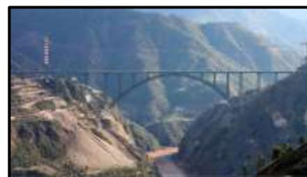
Located in Reasi district, J&K, the Chenab Bridge is part of the Udhampur-Srinagar-Baramulla Rail Line. Built 359 m above Chenab River, it is the world's tallest railway arch bridge. Spans 1,315 m; designed to withstand winds (266 km/h), earthquakes (magnitude 8), and -20°C temperatures. Executed by Konkan Railway, Afcons, VSL India, Ultra Engg. Supported by SAIL, IISc, IITs, DRDO, and Swiss firm Mageba.
